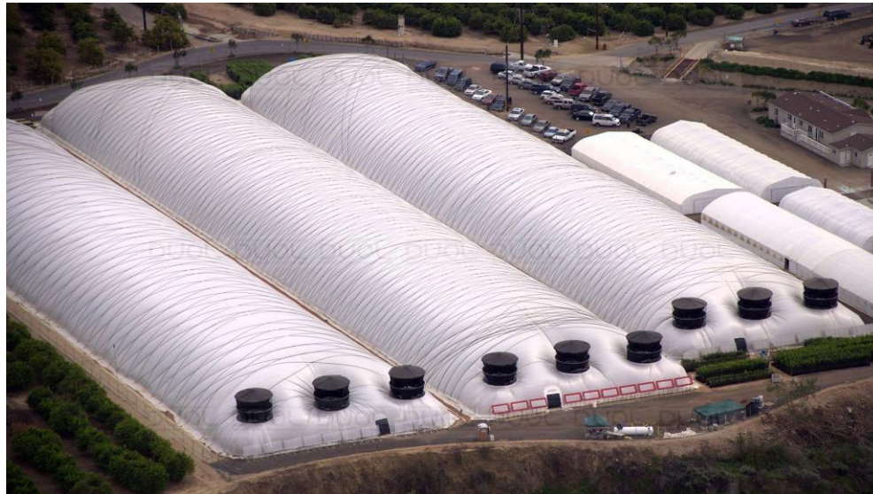
GreenDome, view from outside.
