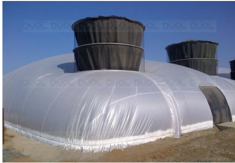
Innovative „WindCatcher Tower“
